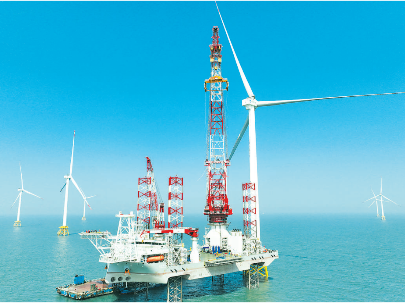
The photo shows part of an offshore wind turbine unit and a 2,000-ton self-elevating offshore wind power installation platform on the waters of southern Fujian in southwest China, January 13, 2026. (PHOTO: XINHUA)
