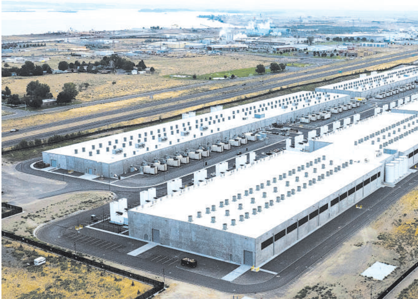
The Amazon Web Services data center in Boardman, Oregon, U.S. (PHOTO: VCG)
