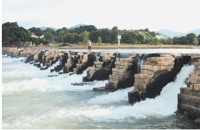
The Mulanbei Water Conservation Project in Mulan, a village southwest of Putian city of Fujian province in southeast China, has been in operation for nearly 1,000 years. (PHOTO: VCG)
