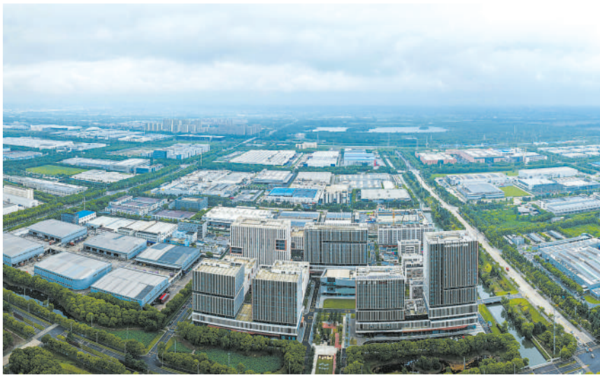
An aerial drone photo taken on June 24, 2026 shows a view of the Sino-German industry-education integration industrial park and surrounding areas in Taicang, east China's Jiangsu province. (PHOTO: XINHUA)
