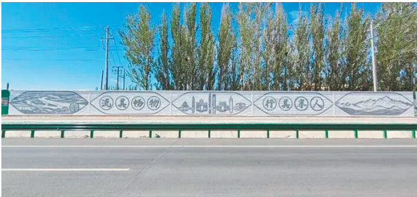
A 50-meter-long, three-meter-high noise barrier built by 3D printing technology in Ningxia Hui autonomous region. (COURTESY PHOTO)
