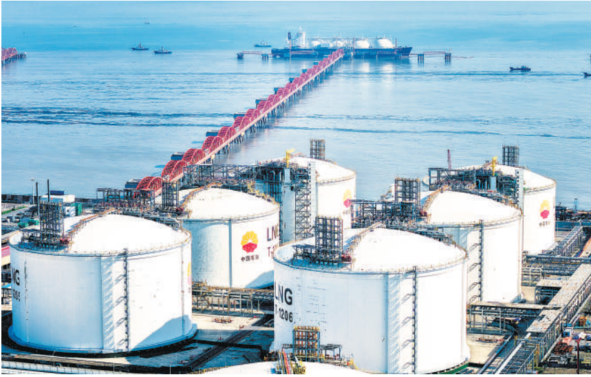
The storage tank area and receiving terminal of an LNG receiving station at Yangkou Port in Rudong, Jiangsu province. (PHOTO: XINHUA)
