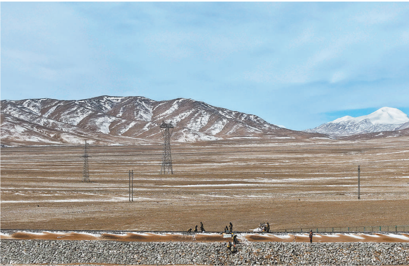
Staff from China Railway Qinghai-Xizang Group Co., Ltd. carry out maintenance work on the Qinghai-Xizang Railway in the heart of the Kunlun Mountains in February, 2026. (PHOTO: XINHUA)
