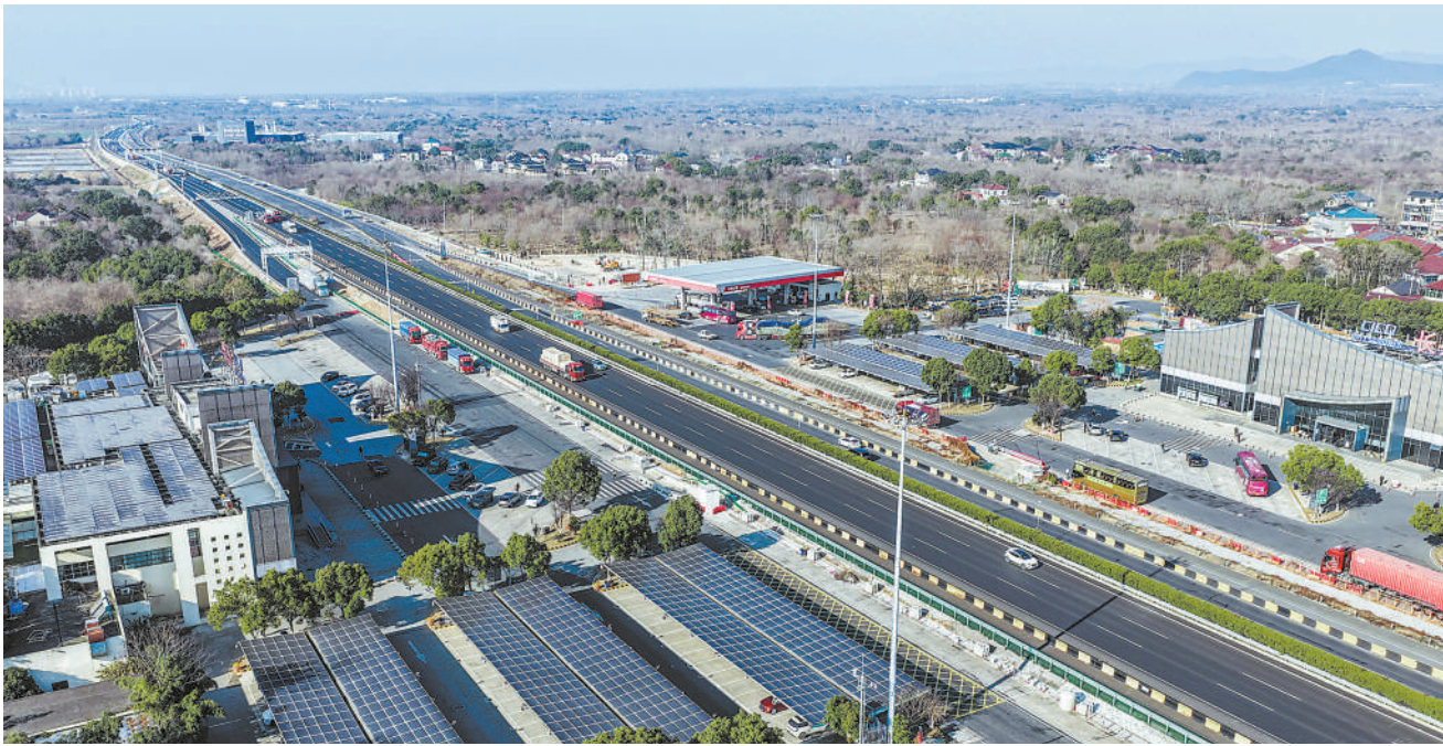
Beneath the photovoltaic panels is the upgraded charging station at the Changxing Service Area on the G50 Shanghai-Chongqing expressway, January 7, 2026. (PHOTO: XINHUA)
