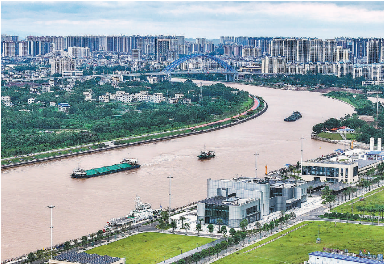
The Pinglu Canal in Guangxi Zhuang autonomous region becomes operational on September 16. (PHOTO: XINHUA)
